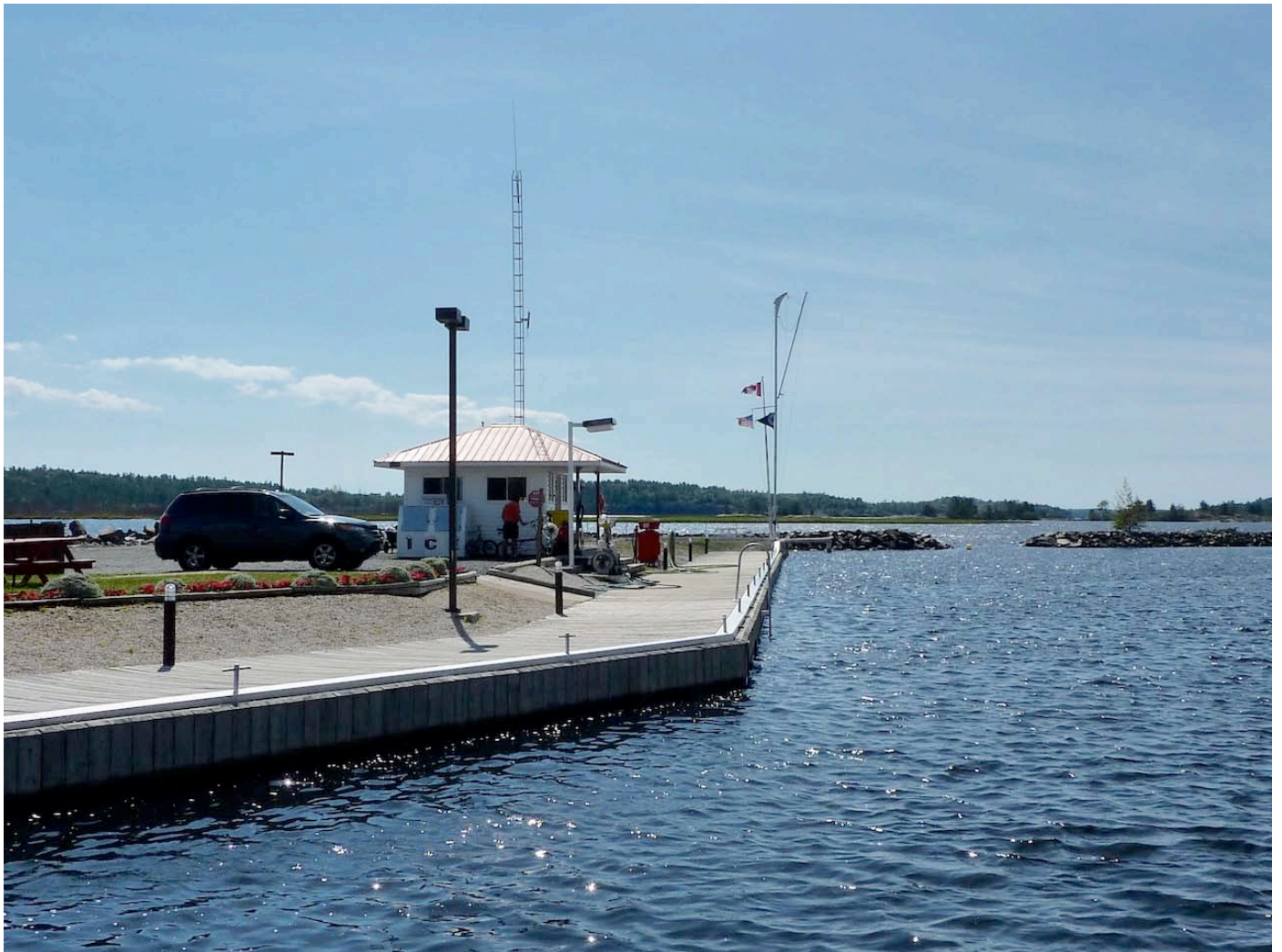
We're off- through that little gap in the breakwall.
